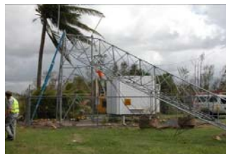
A failed communication tower in Silkwood one of the results of Cyclone Larry (see cover story)
