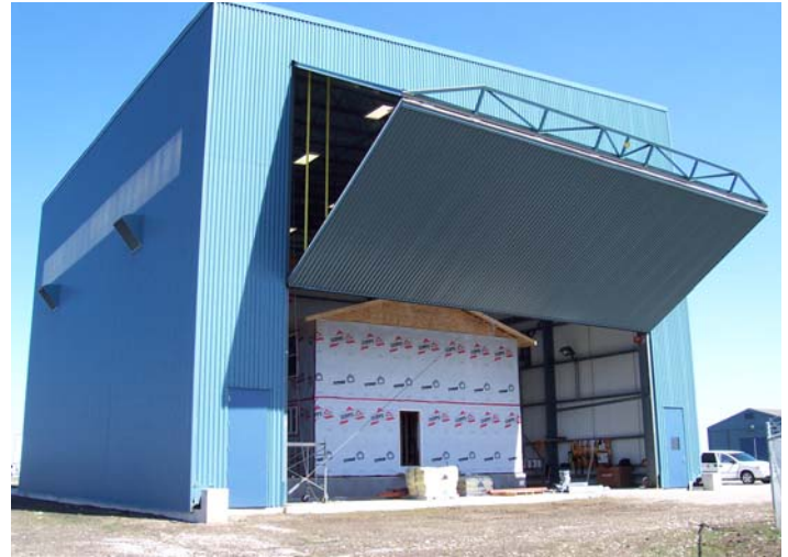
Figure 1. The hangar building covering the first house specimen (under construction).
