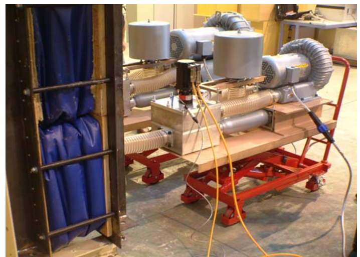
Figure 4. Photograph of two prototype pressure loading actuators connected to the (blue) pressure boxes, the flexible membranes connecting the PLAs to the house surface to allow the pressures to be applied.
