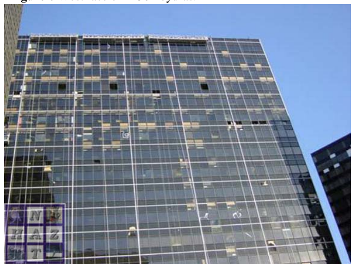
Figure 6 West face of 1250 Poydras.
