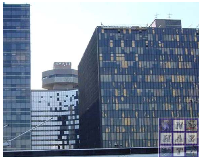
Figure 2 Damage to Hyatt Regency Hotel and Amoco Building as seen from the roof of City Hall
