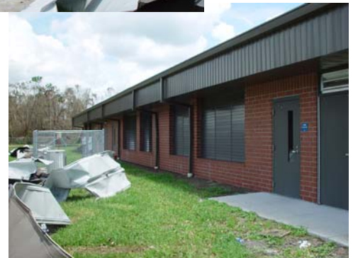
Adjacent classroom building that was built to EHPA criteria was undamaged
