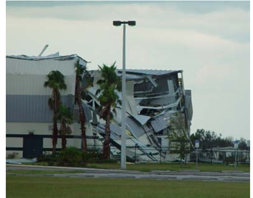
Significant end wall failure at the newly constructed Turner Agri-Civic Center shelter in Arcadia Florida during Hurricane Charley
