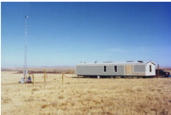
Figure 1. Manufactured home tested at field site near Arlington, WY
