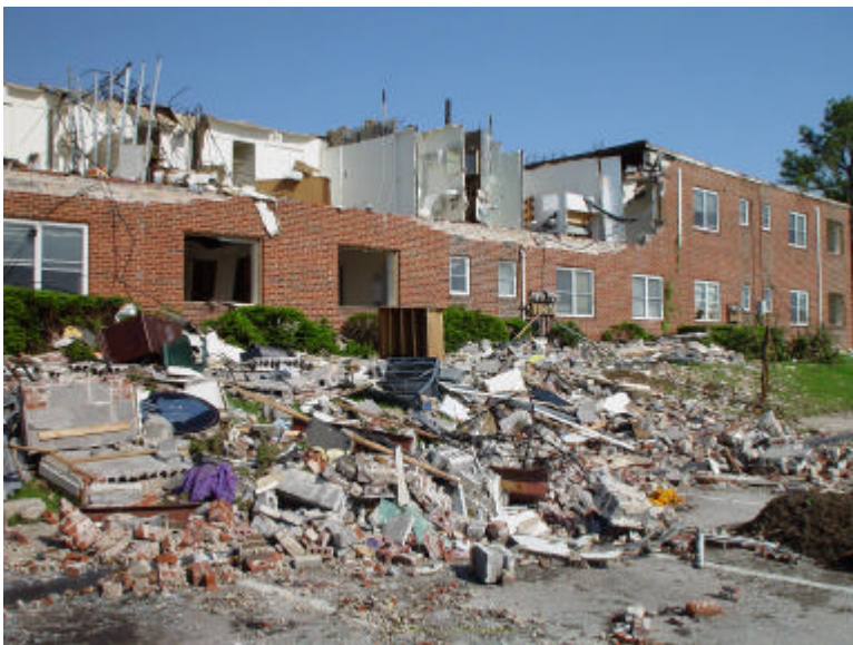
Figure 16 Damage to William Jewell College dormitory
