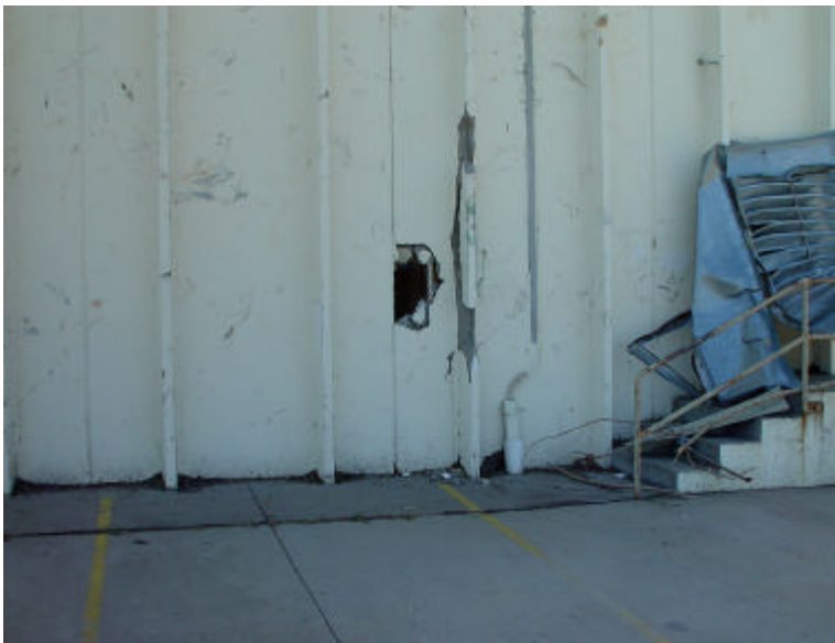
Figure 19 Three-inch thick concrete wall panel was penetrated by a UFM (unidentified flying missile)
