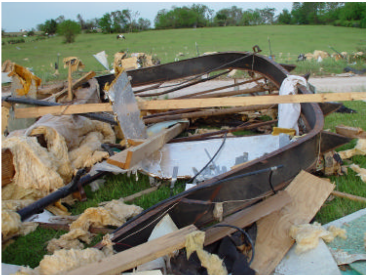
Figure 3 Undercarriage of a manufactured home approximately 100 feet from its original location
