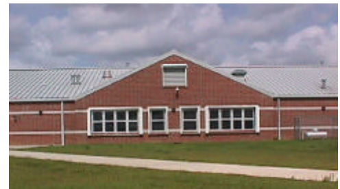
Figure 1. Typical retrofitted school building with window and lower protection
