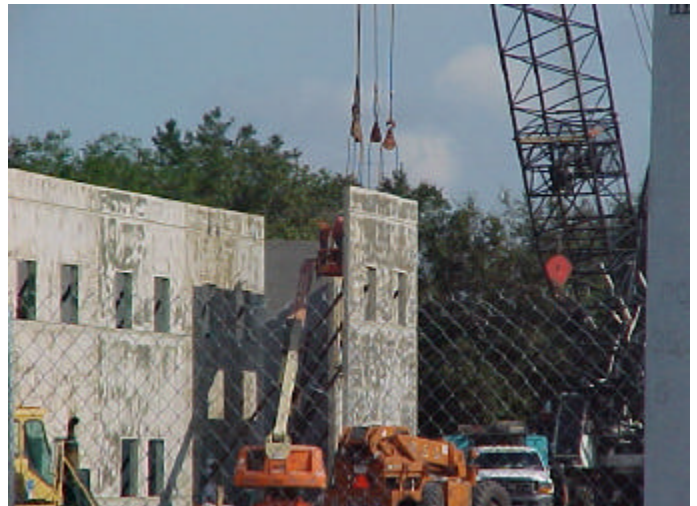
Figure 2. New school facility being constructed to the public shelter design criteria
